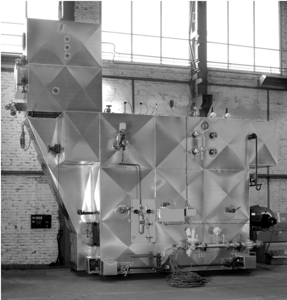
Fig. 2-4: Corner tube boiler
