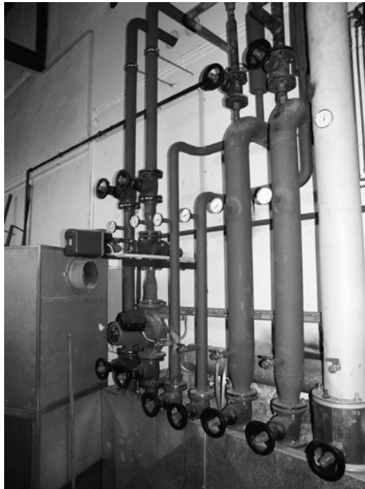
Fig. 4-8: Uninsulated indoor pipes
